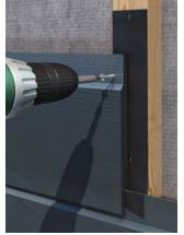
down to size, take into consideration a 10 mm ventilation outlet gap between the top edge of the board and the roof line. It will need to be fixed with the Hardie™ Plank screw and then the head, filled and painted. Alternatively, use a Hardie™ Plank coloured screw.
