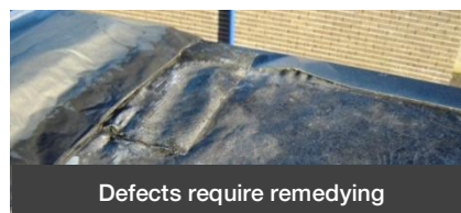
PVC Single-ply roof
