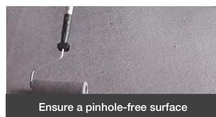
Wetting through the fibreglass CSM
